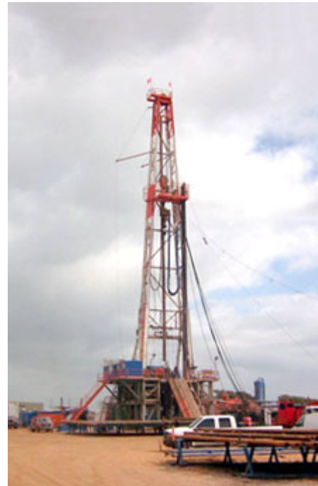
Drilling Webb-1 Well
